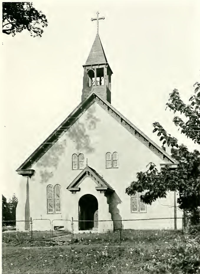
CHRIST, BUILT ABOUT 1735 PORT REPUBLIC, CALVERT COUNTY
